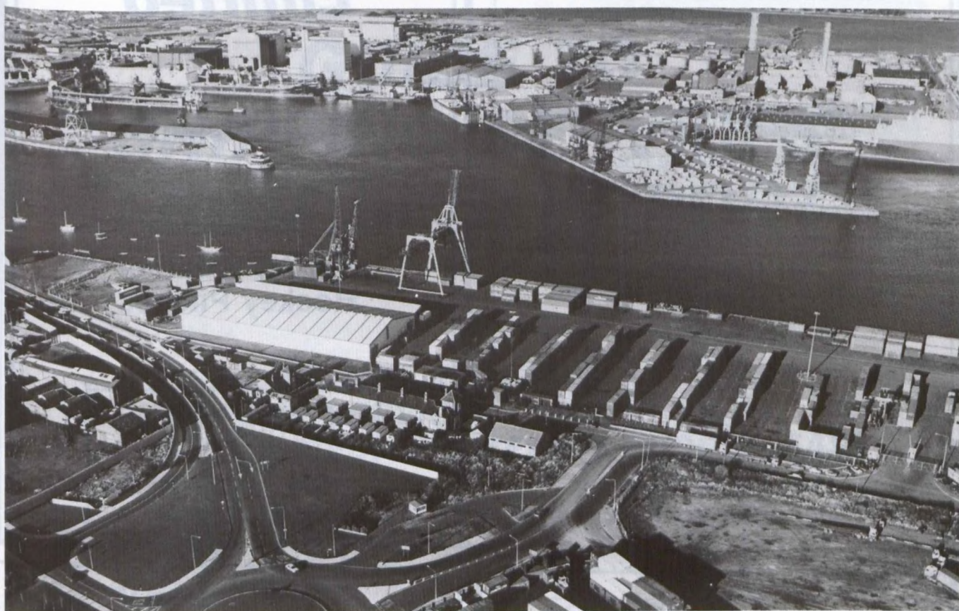
Aerial view of Dublin Port - Southside.
