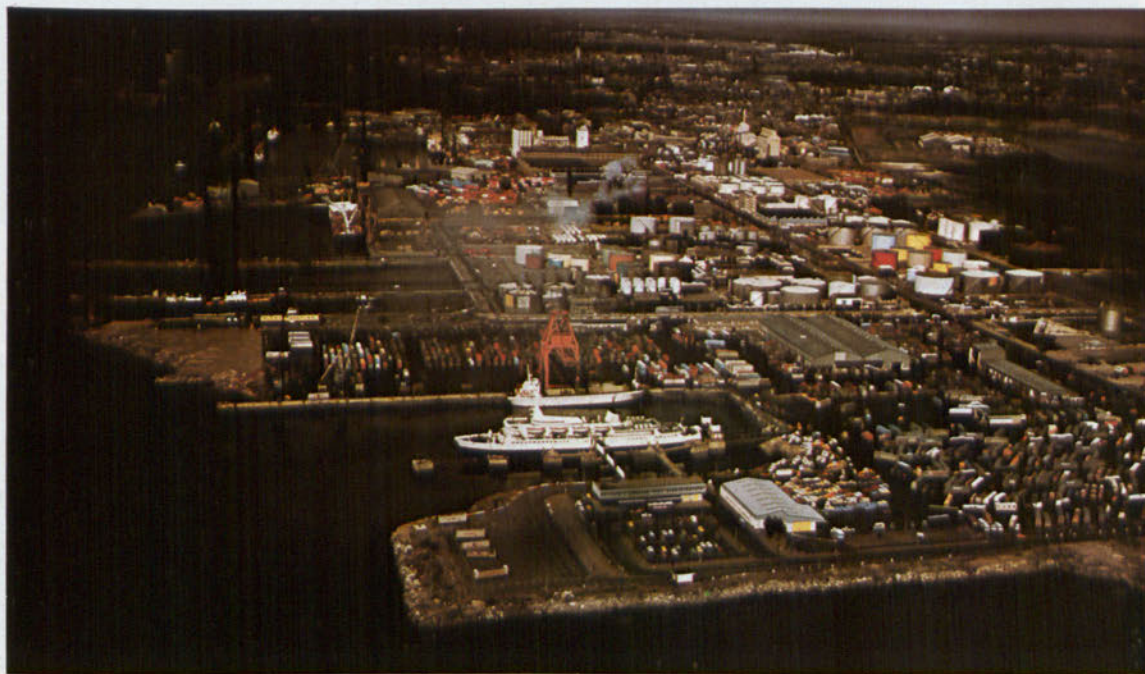
General view of the port with No. 1 Ro/Ro Terminal and B+I Line Freight Terminal in the foreground.
