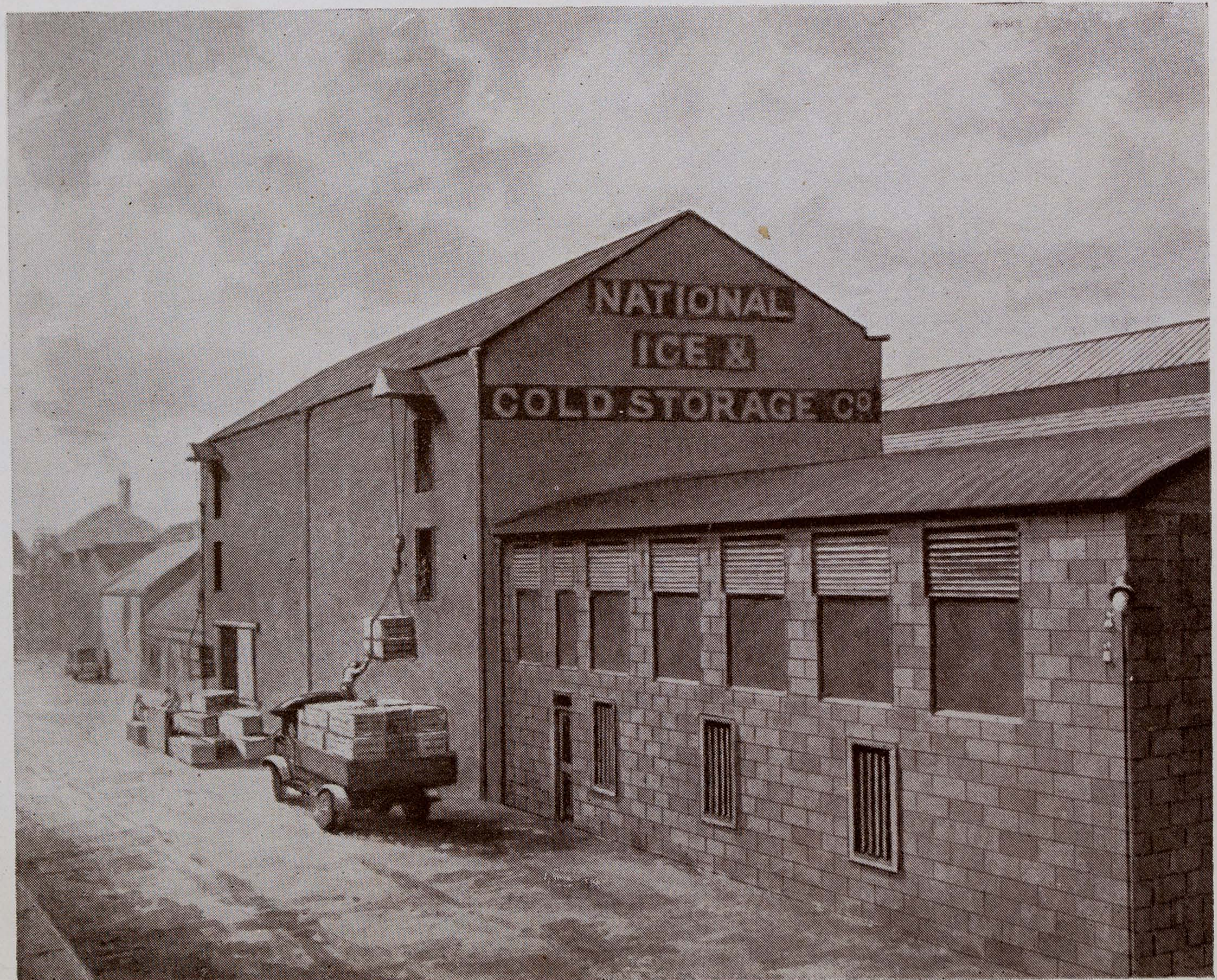
The National Ice and Cold Storage Co.'s Cold Stores, 28 Sir John Rogerson's Quay.
